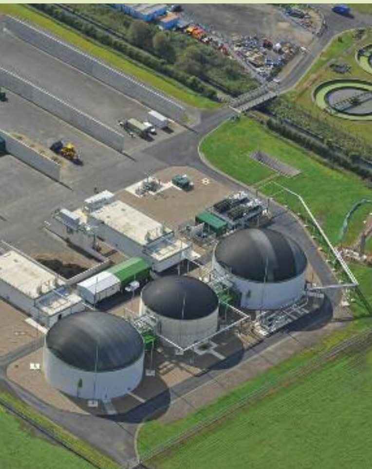
The Severn Trent AD Plant at Stoke Bardolph
